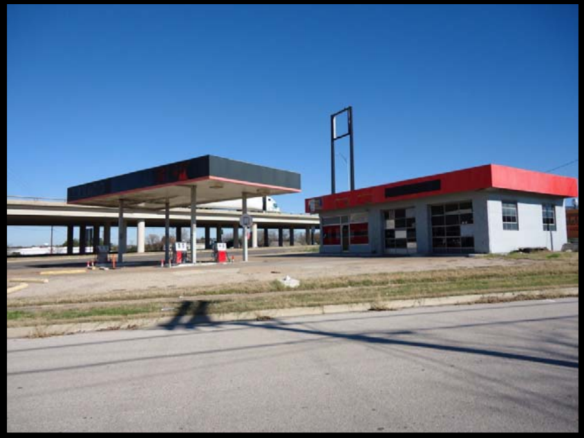
Site: Developed with Unoccupied Gas Station - Looking North (NS)
